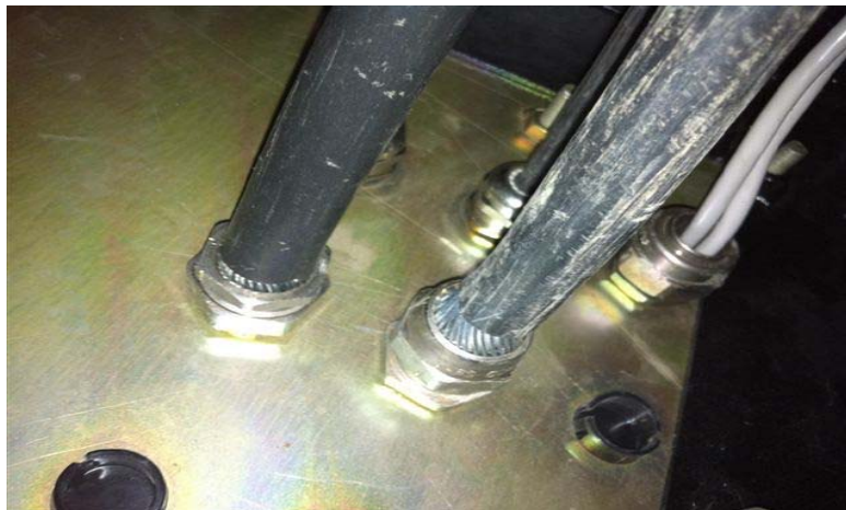
Figure 3: Cabinet gland plate (bottom/top of the cabinet)
