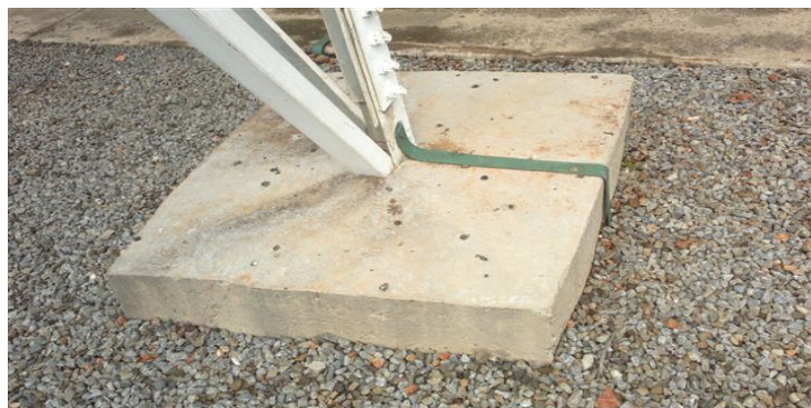
Figure 2: Tower leg grounded on the tower ring
